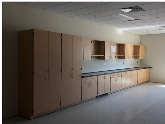
Casework install at WPA
