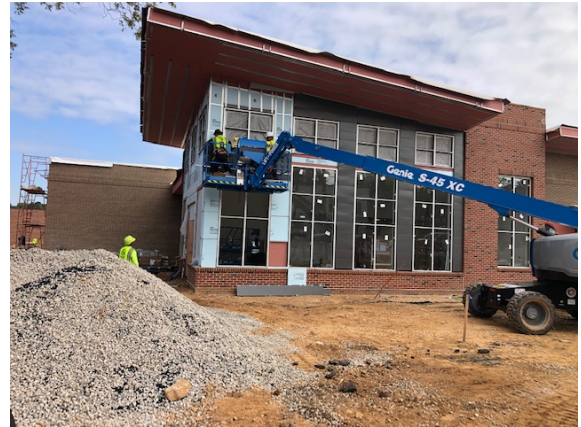
Metal Panel install at South Elevation at YMCA
