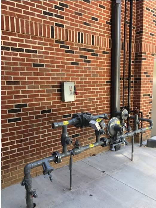
Gas meter installed at WPA
