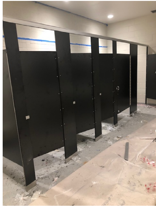
Toilet partition install at WPA
