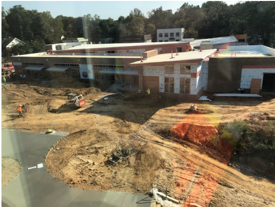
North side of the YMCA
